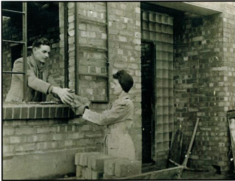
Photograph of workers building one of the houses on the estate, possibly Prince Charles Avenue, late 1940s
